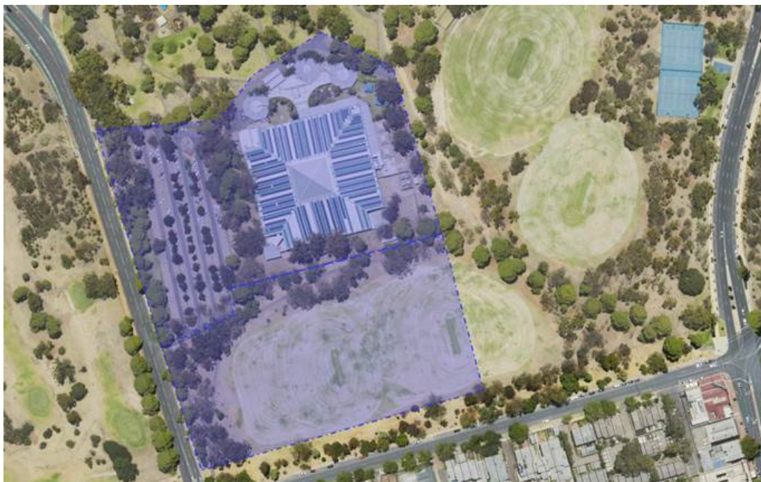
Image 3 – Temporary Works Compound: (Stage 2 – 35,000 sqm)
